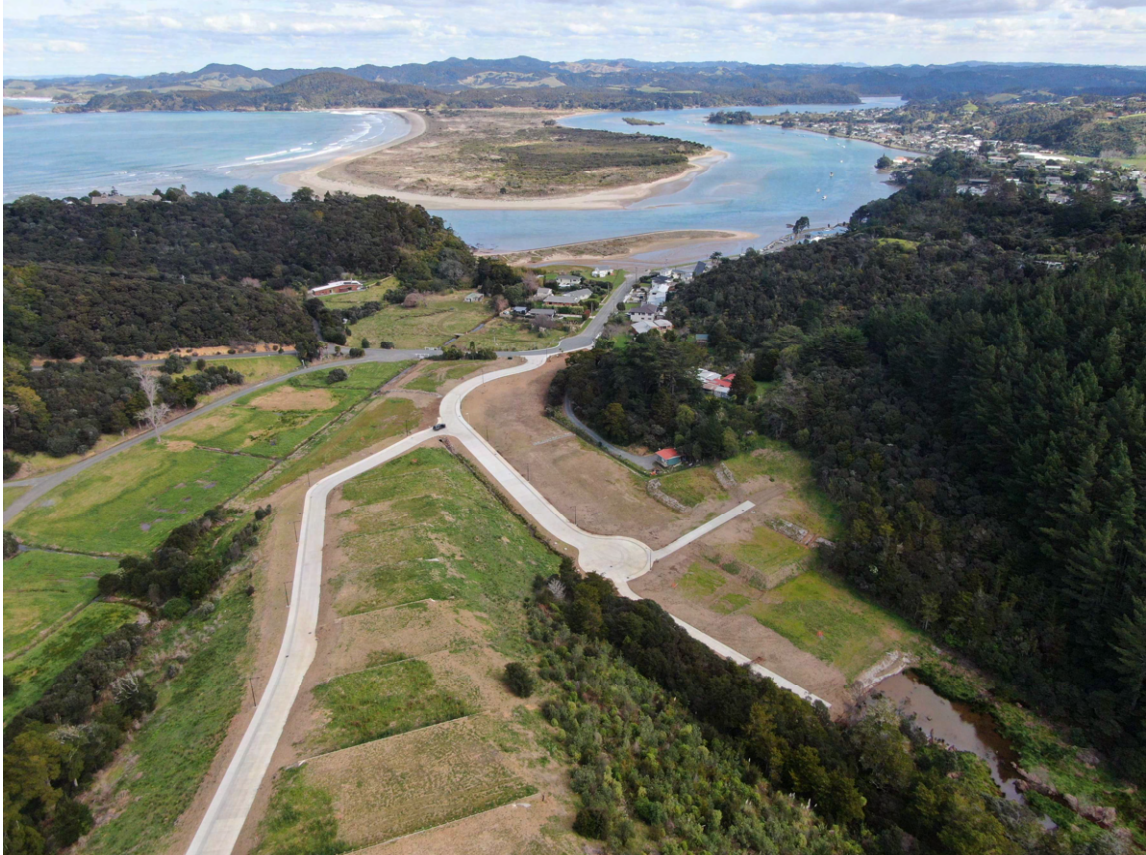
Te Maika Road Core Engineering Solutions Ltd
